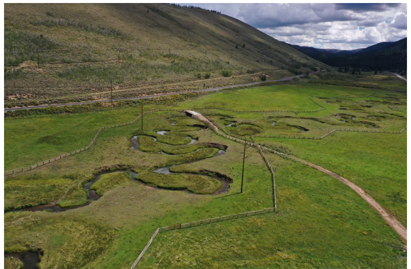
Figure 5 Oblique Imagery showing the construction of the new riparian exclusion fence along Mud Creek.
